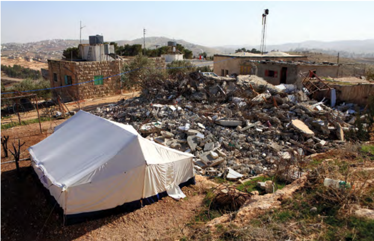
Ruins of a Palestinian house in the village of Al Nu'man, east of Beit Sahour. © Activestills/Anne Paq, December 2010
