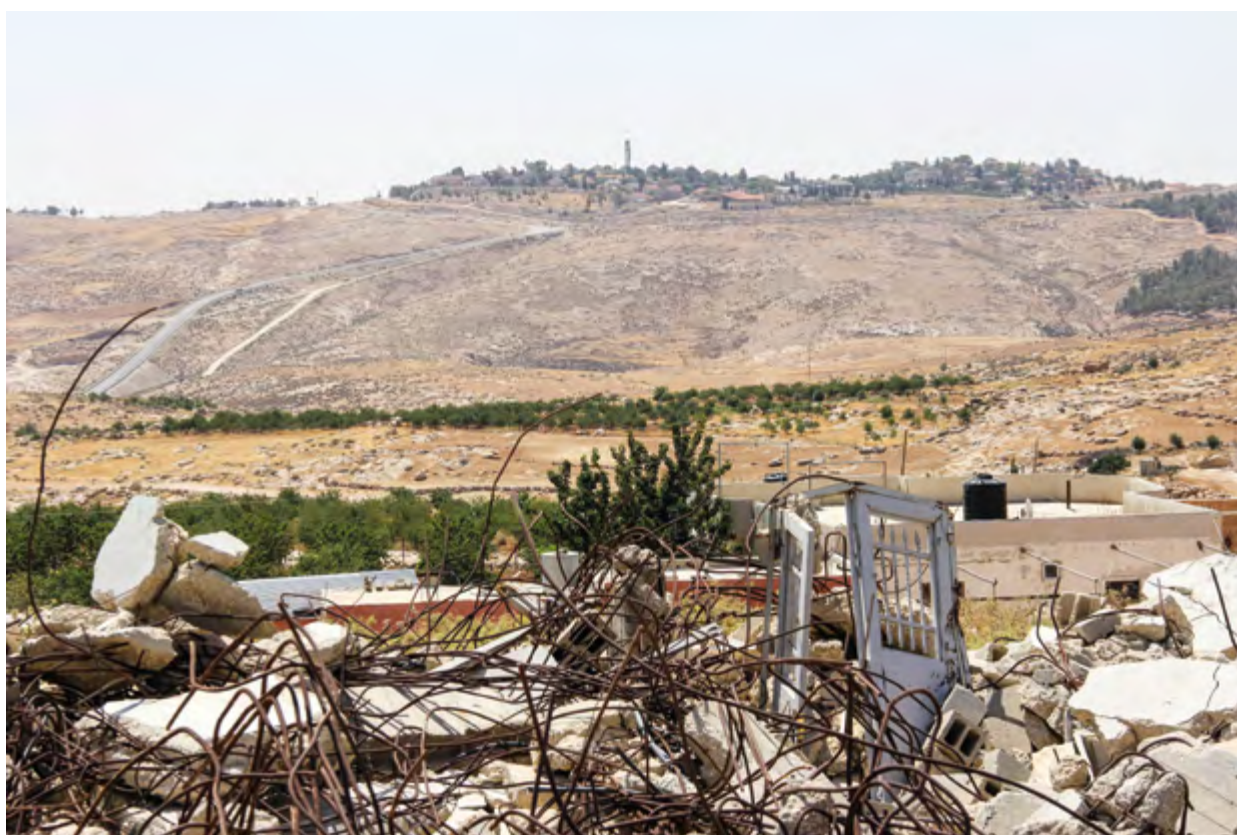
Ruins of a Palestinian house in the village of Ad Deirat, south of Hebron and east of Yatta in an Israeli-controlled area. The house was demolished in 2013 and its residents forced to move to Yatta. The settlement of Carmel can be seen in the background. Credit: H el ene Bohyn, June 2015.
