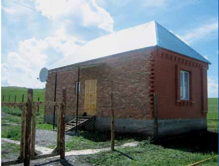
New housing for a displaced family from Chechnya who opted to stay in neighbouring Ingushetia, July 2007. Photo: Nadine Walicki, IDMC
