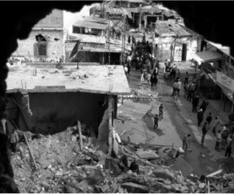
Palestinians inspect the rubble of their houses after they were demolished by Israeli bulldozers during a raid in Rafah Photo: Reuters/Ibrahim Abu Mustafa
