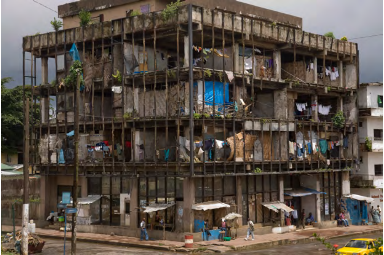
Abandoned office building in Monrovia, hosting urban internally displaced persons. Photo: Christopher Herwig, June 2006
