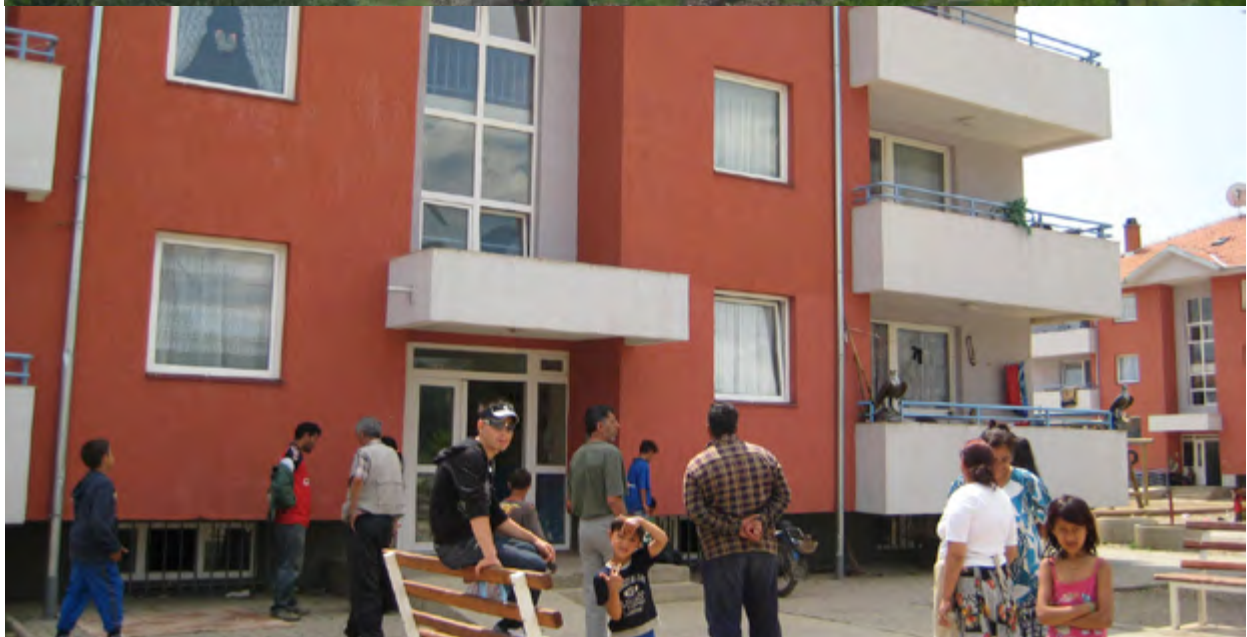
View of the destruction of Roma Mahalla after the conflict, and of a rehabilitated building. Photo: IDMC/B. McCallin, May 2009
