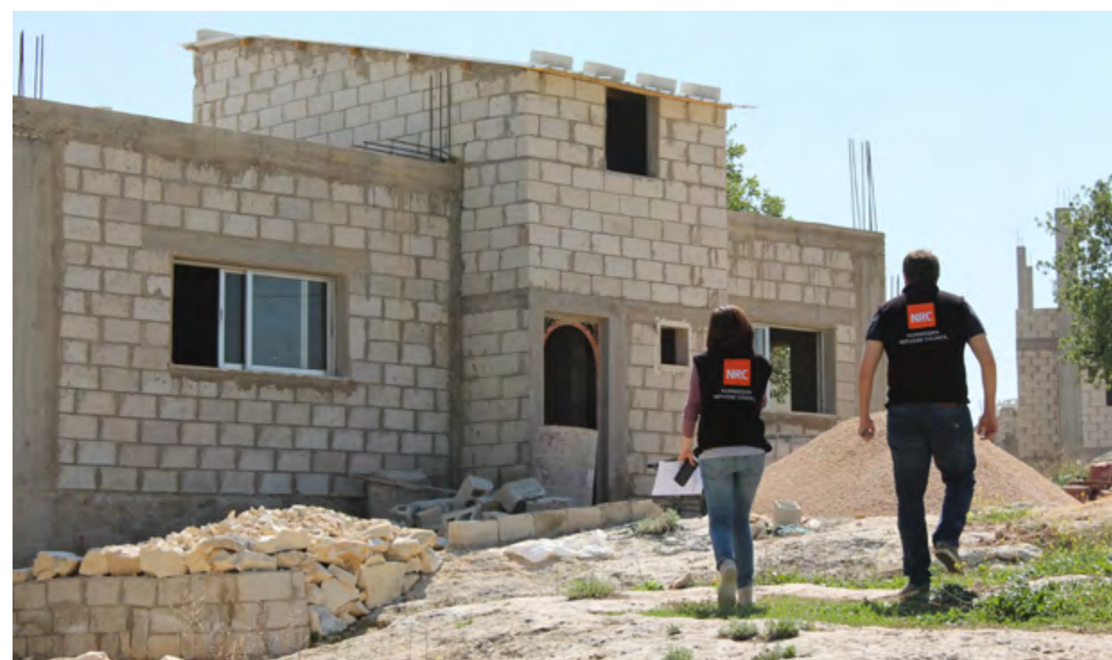
NRC engineers assess construction works for Syrian urban refugees in Jordan. Photo: NRC Jordan/Rawan Baybars, March 2014
